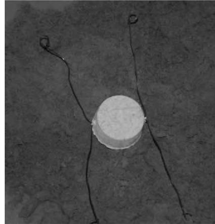
*Fig. 2. Sacrificial zinc anode installed*
