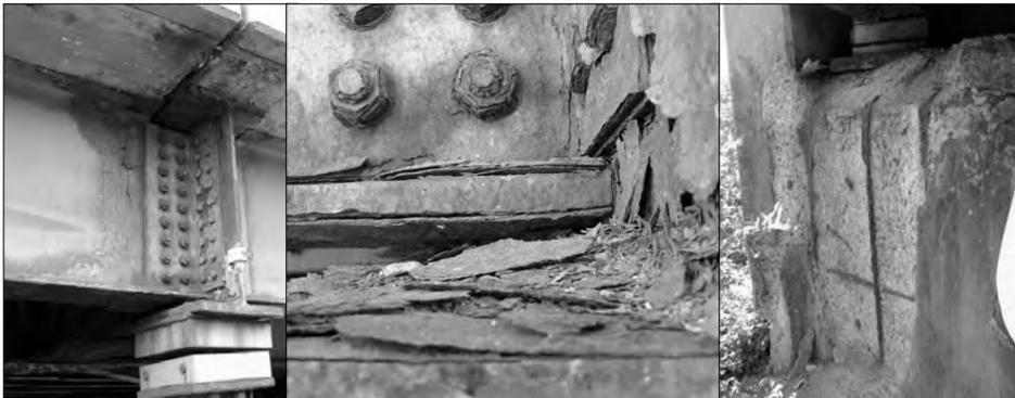
*Fig. 1. Left: Steel corrosion below transverse joints. Centre: Delamination and pitting corrosion. Right: Freeze-thaw attack in abutment.*
