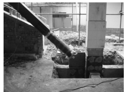
Fig. 1 Elevation of the damaged Primary School Fig. 2 Construction of the retrofitting damper bracings
