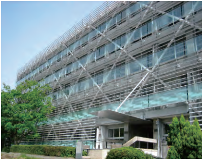
Fig. 3: Retrofit with energy-dissipating grid-skin
