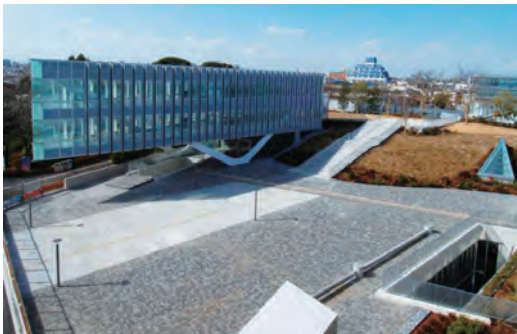
Fig. 1: Steel grid-skin supported by diagonals
