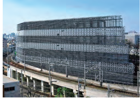
Fig.4: Grid-skin supporting solar cells
