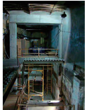
Fig. 3: View of Lateral Stability Frame during construction above the new escalator wellway
