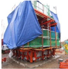
(a) Completed assembling of slip form
