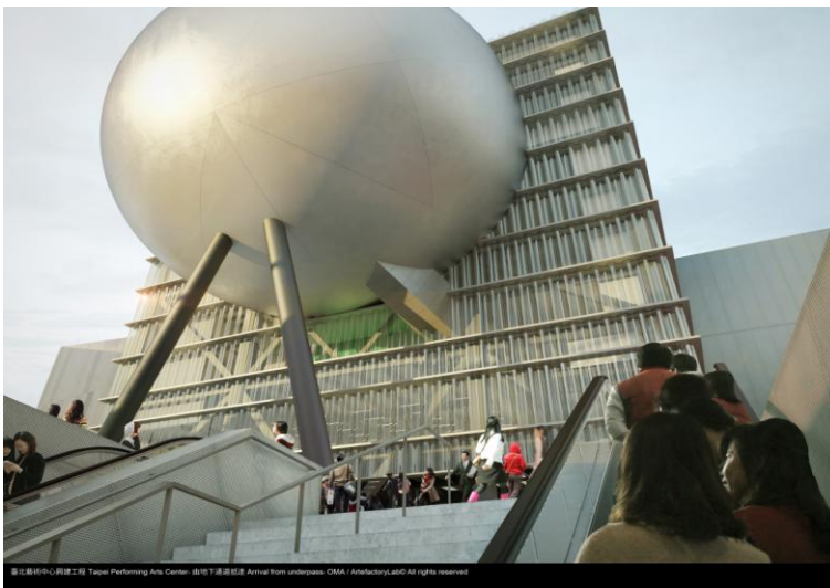
Fig. 3 The corrugated glass facade of the Taipei Theatre.
