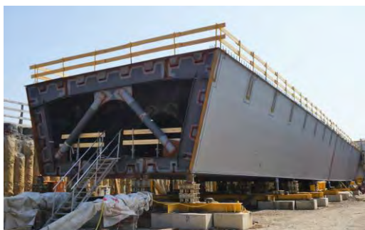
Figure 1. Design variants of tubular bracings inside and outside of box girders of the German bridges Heidingsfeld (left) and Hochmosel (right)
