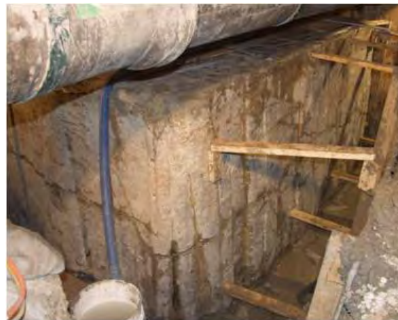
Figure 2. Cracking on side surfaces.
