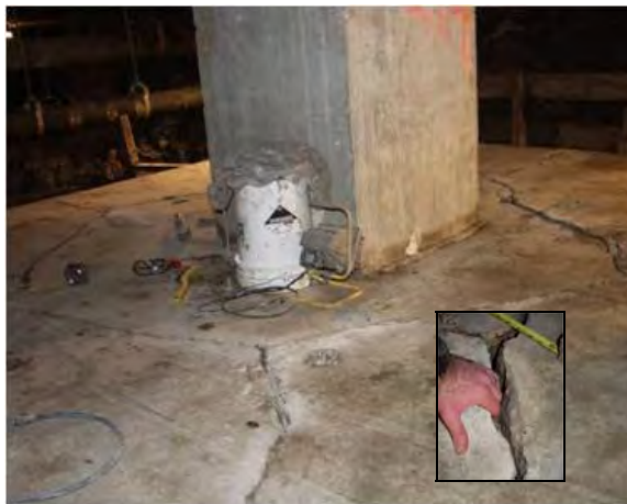
Figure 1. Typical cracking on top of pile cap.
